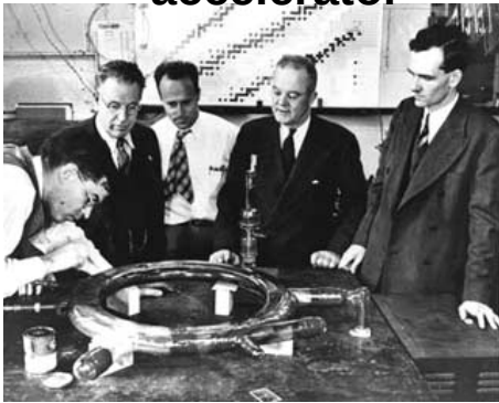
Vacuum chamber of GE synchrotron
