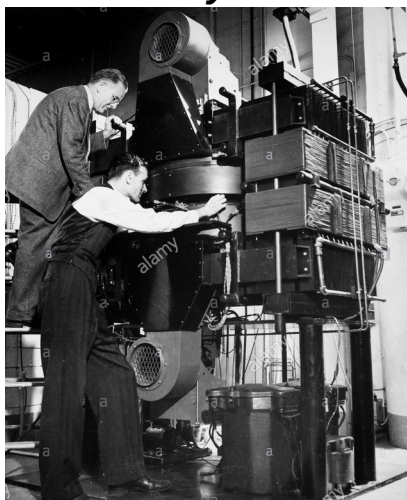
Vacuum chamber of GE synchrotron
