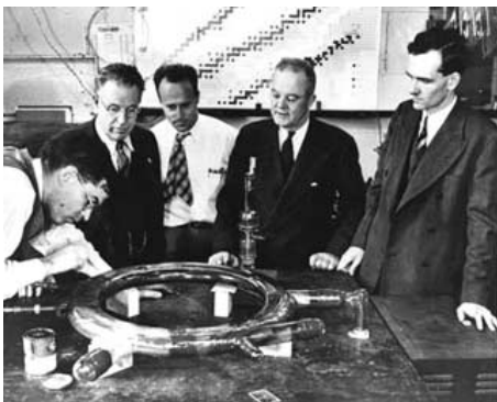
Vacuum chamber of GE synchrotron
