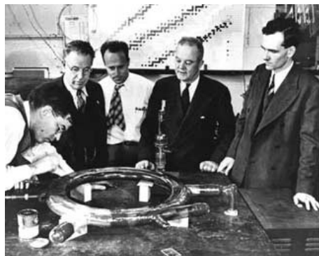
Vacuum chamber of GE synchrotron
